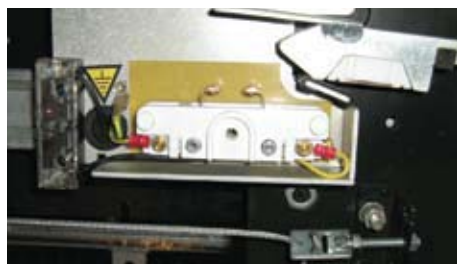
EXAMPLES OF INCORRECT LIFT INSTALLATIONS DETECTED IN VICTORIA – EXPOSED CONNECTIONS AND INCORRECT CABLE IDENTIFICATION.
